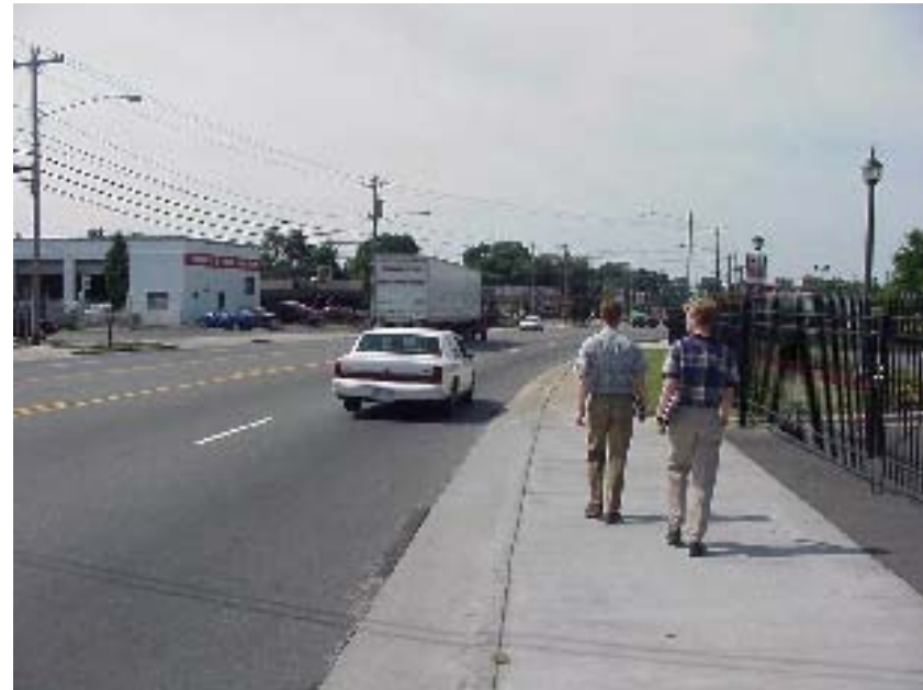
The existing land development pattern and streetscape in the Commercial District is designed to serve the automobile.
