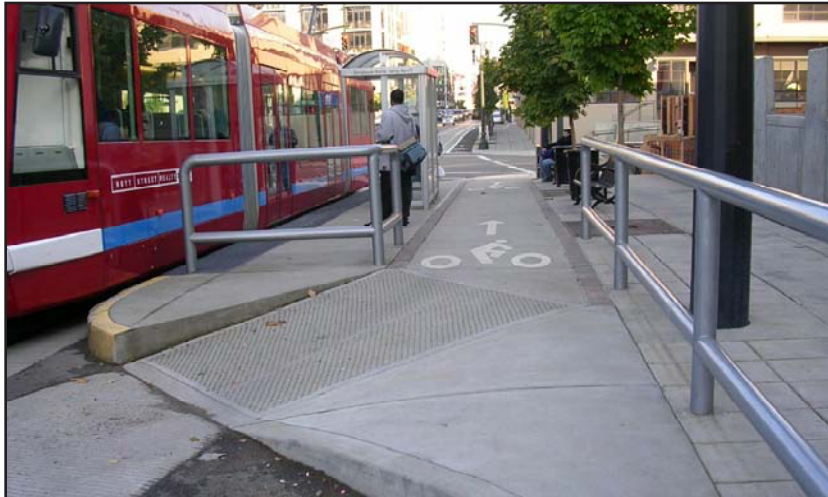
The public sector will be responsible for most of the improvements to transit and infrastructure.
