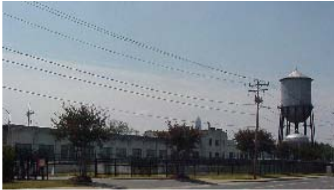
Vest Water Works
