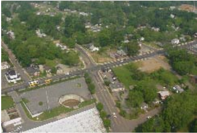
Intersection of Beatties Ford Road and Oaklawn Ave./Booker Ave. before the road improvement project in 2002.
